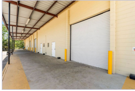
Covered loading dock
