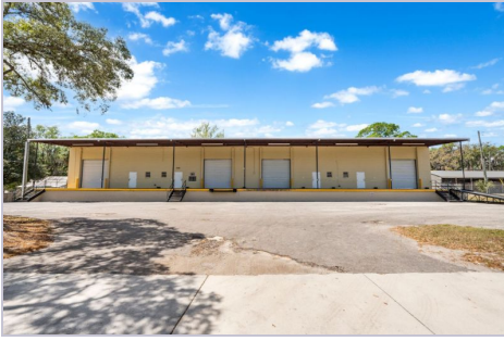
Front elevation: four roll-up doors, stairs, truck ramp
